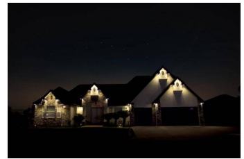
Warm-white roofline and gables
